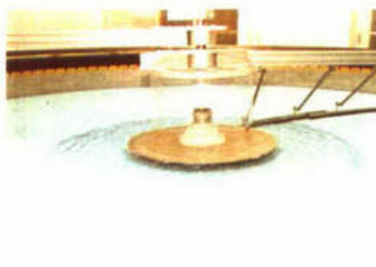
b) Concentric Inlet/Sludge Hopper device
