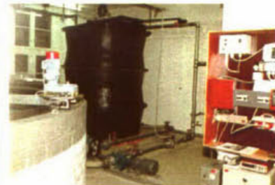
i) In the Foreground the Drive of the Scraper moving on a Circular Rail. In the Background the Stirring Tank
