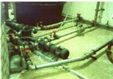
h) Pipe Network for Inflow and Recirculation
