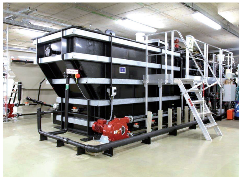
CENIRELTA Mainstream Anammox demonstration reactor
