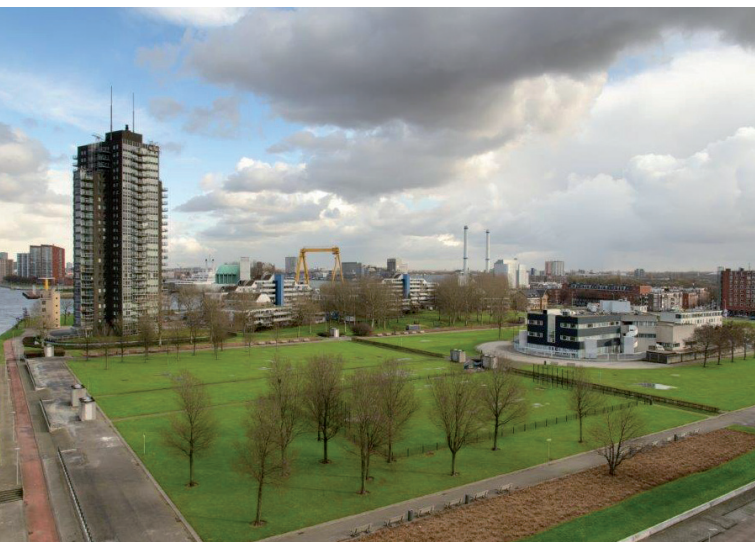
WWTP Dokhaven, Rotterdam, The Netherlands
